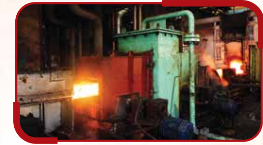
WALKING BEAM TYPE BILLET REHEATING FURNACE
