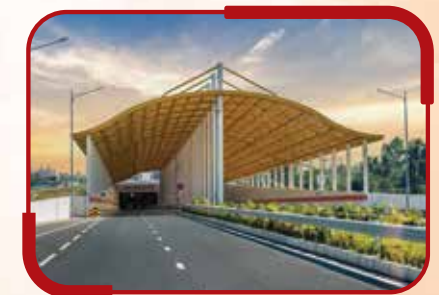
Karnaphuli Tunnel Project
