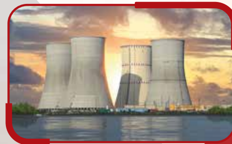
Rooppur Nuclear Power Plant Project
