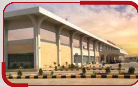
Osmani International Airport Project
